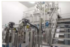
Equipment to mix chemicals
